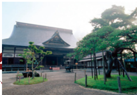
中尊寺本堂 The main building of Chusonji
